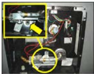
Water Heater Drain Plug Location
